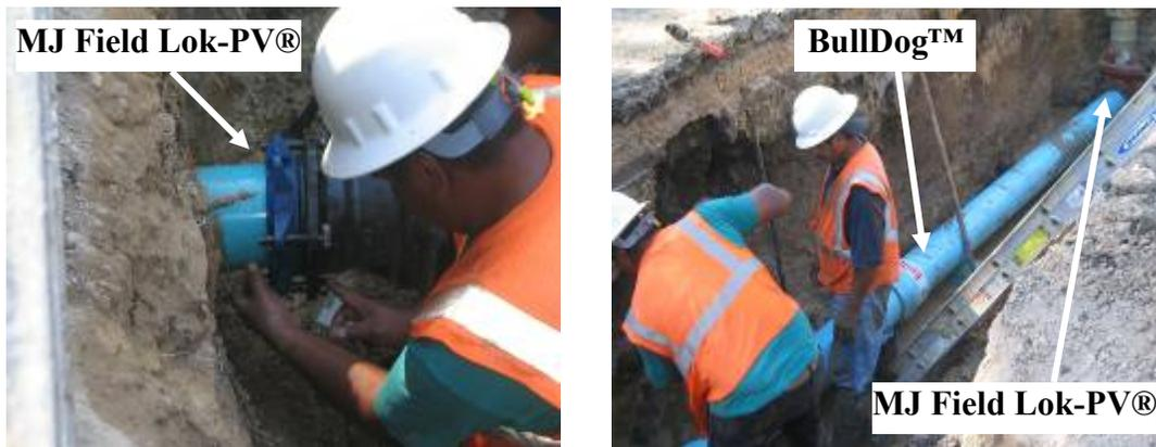
Figure 11: Joint Restraints at Tie-In A
