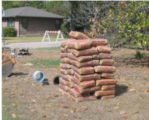
**Figure 13: Concrete at the Job Site that was Unused for Thrust Blocks**
