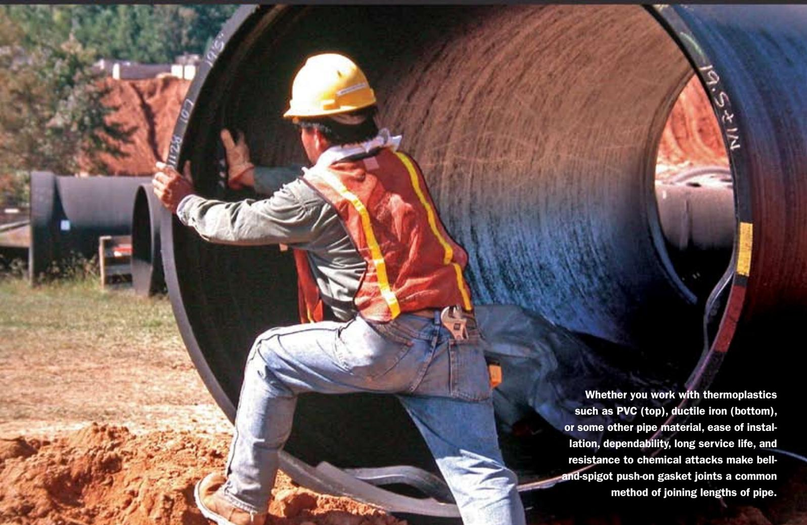
Whether you work with thermoplastics such as PVC (top), ductile iron (bottom), or some other pipe material, ease of installation, dependability, long service life, and resistance to chemical attacks make bell-and-spigot push-on gasket joints a common method of joining lengths of pipe.
